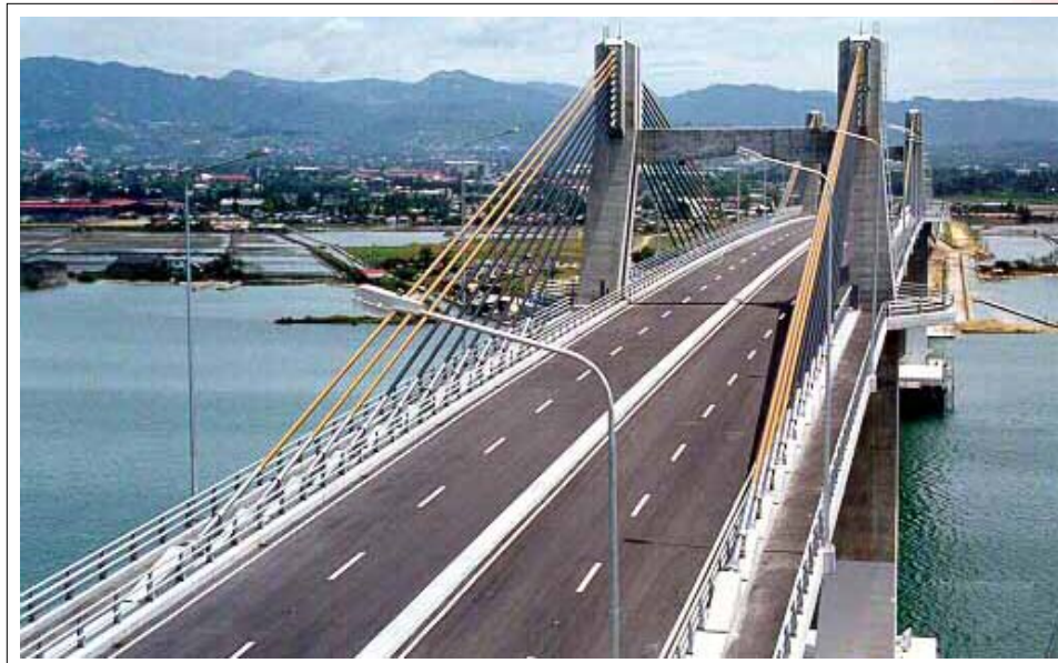
The Second Mactan-Mandaue Bridge has been very effective in reducing traffic congestion and ensuring smooth traffic flow between the islands of Cebu and Mactan
